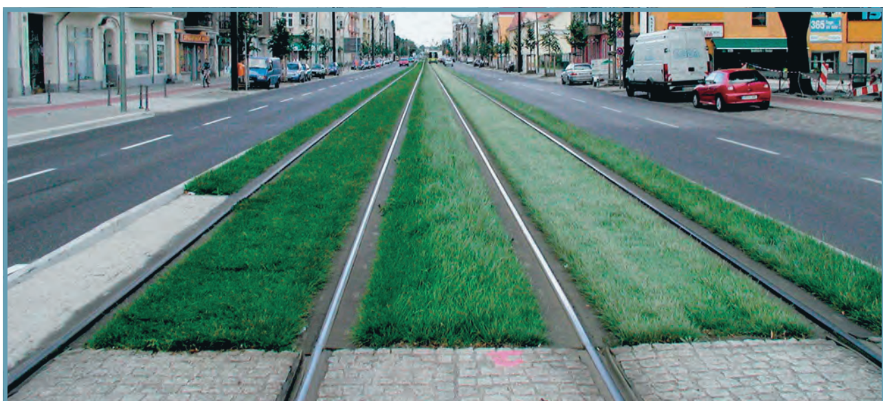
Figure 16: New Standard for Track Construction "Green Tracks" 23
