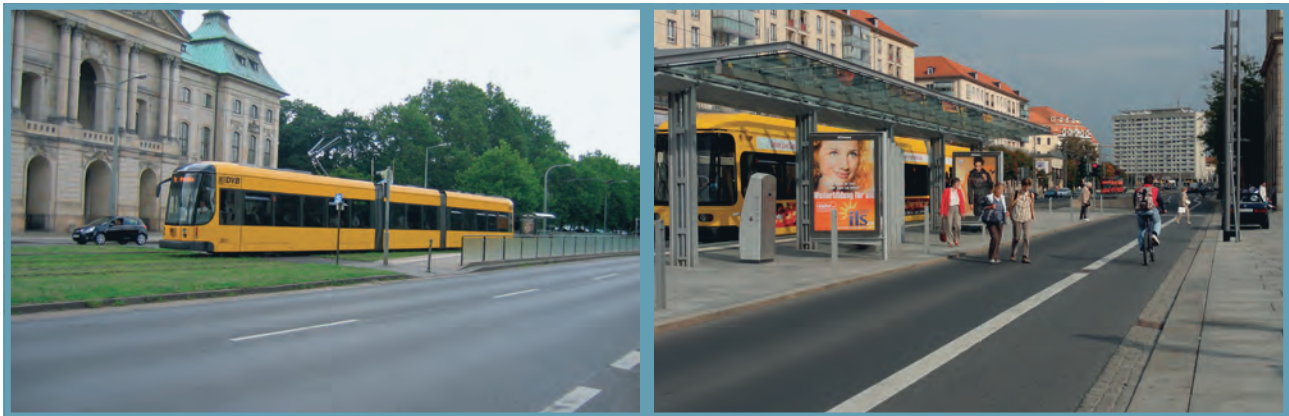
Figure 25: Islands for Tram Stops with or without Barrier on the Road Side 33
