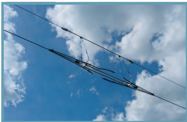
Disconnection of catenaries for a change of the power supply system 13
